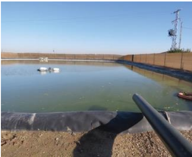
Detail of water inlets to the regulation pond.
